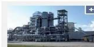
27MW energy system at Kronospan, Brasov
