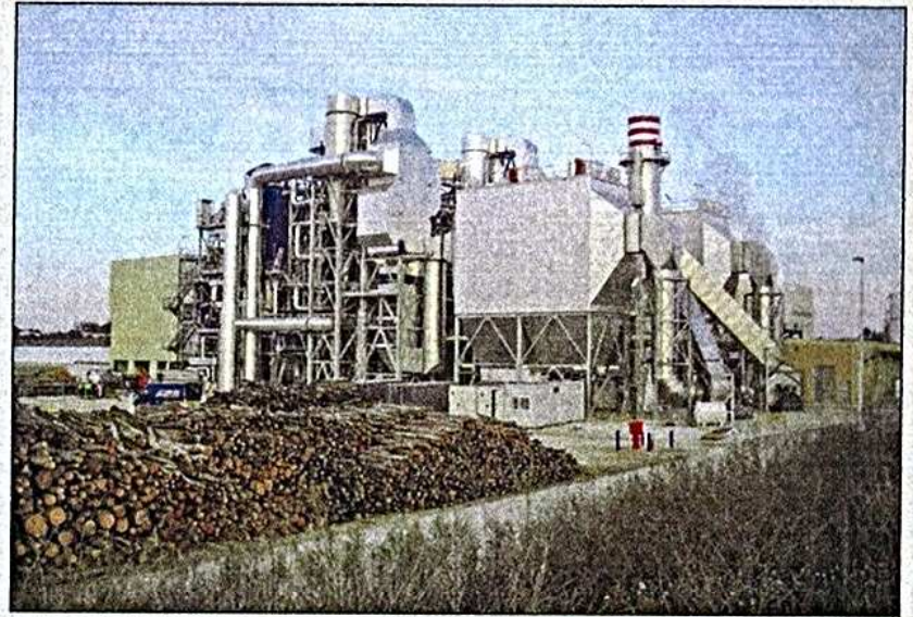
INTEC energy plant in Spain
